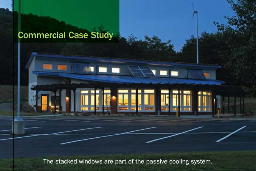
The stacked windows are part of the passive cooling system.
