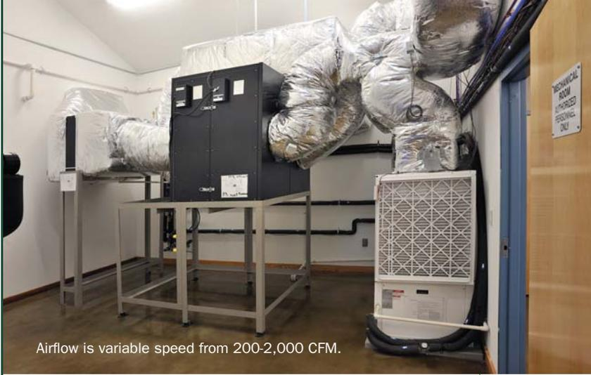
Airflow is variable speed from 200-2,000 CFM.
